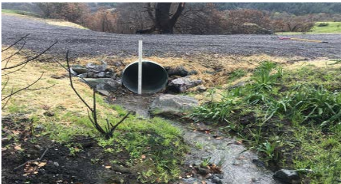
Replaced Culvert at Site 4. Photo by Pacific Watershed Associates.
